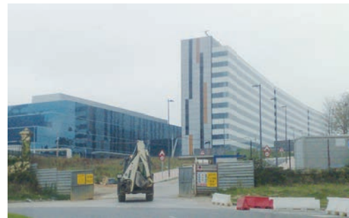
Oviedo Central University Hospital (Asturias/ SPAIN) The air conditioning ducts are constructed with URSA AIR: M2021 Aluminum Roll.
